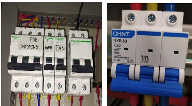
Figure: 4(a) MCB (Schneider & CHINT) MCCB
