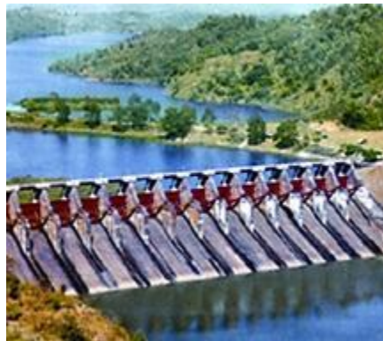
Figure 2.6: Karnaphuli hydroelectric power station
