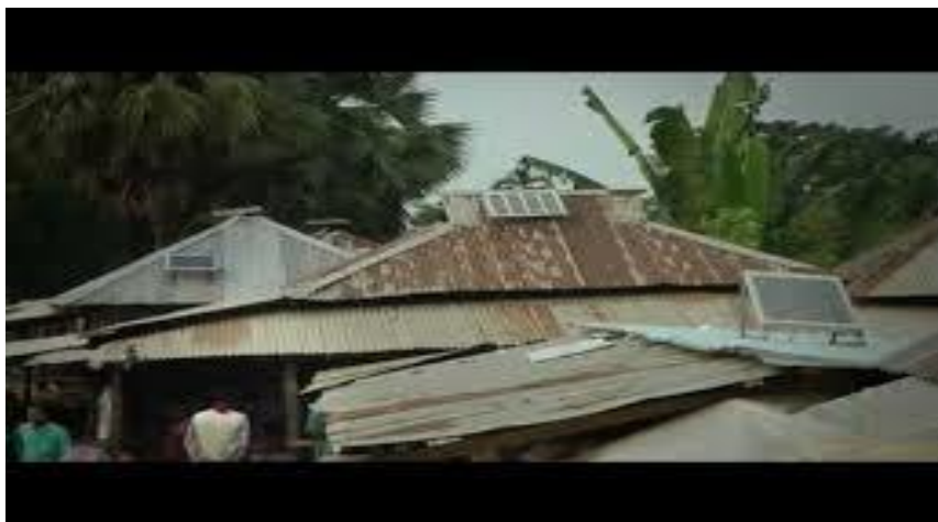
Fig:1 Solar home system of Bangladesh (SHS).
