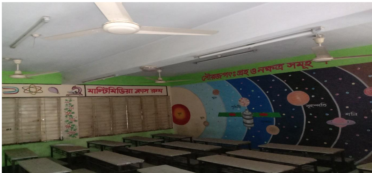
(Image Source: Author.) Load demand image of a one room for government primary school.
