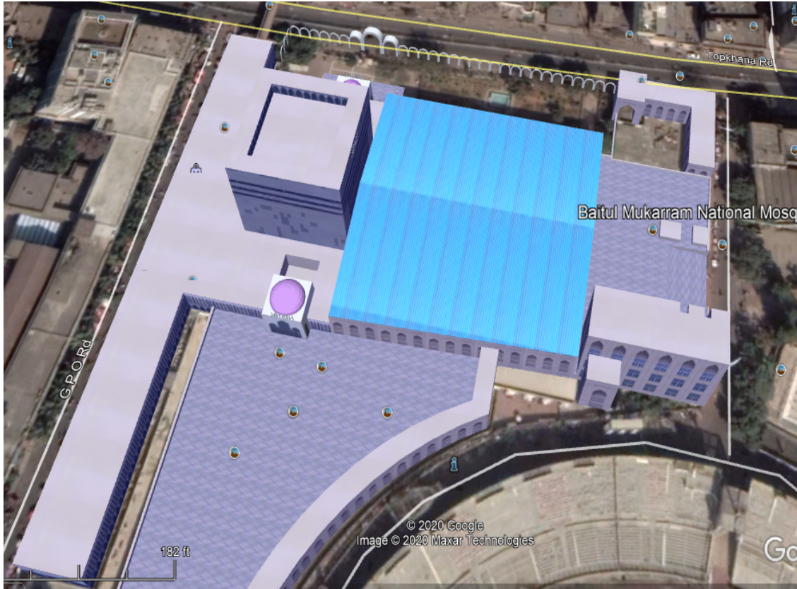
Fig.3. 2: Rooftop area of Baitul Mukarram National Mosque.
