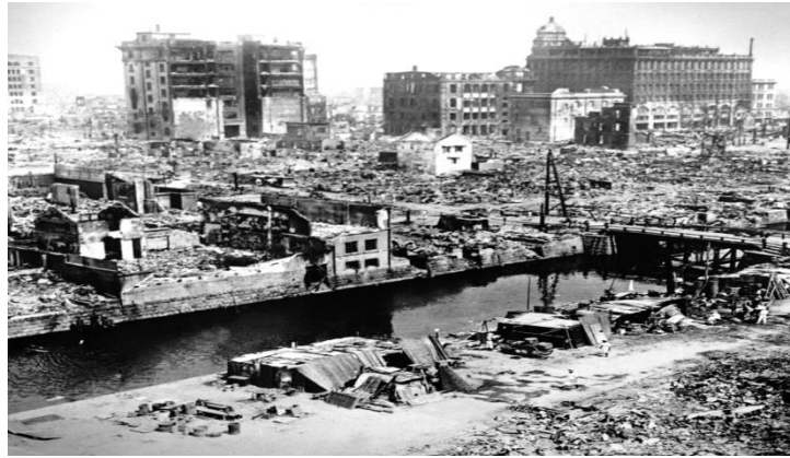
Fig 1.1 The great kanto earthquake in japan 1923.
