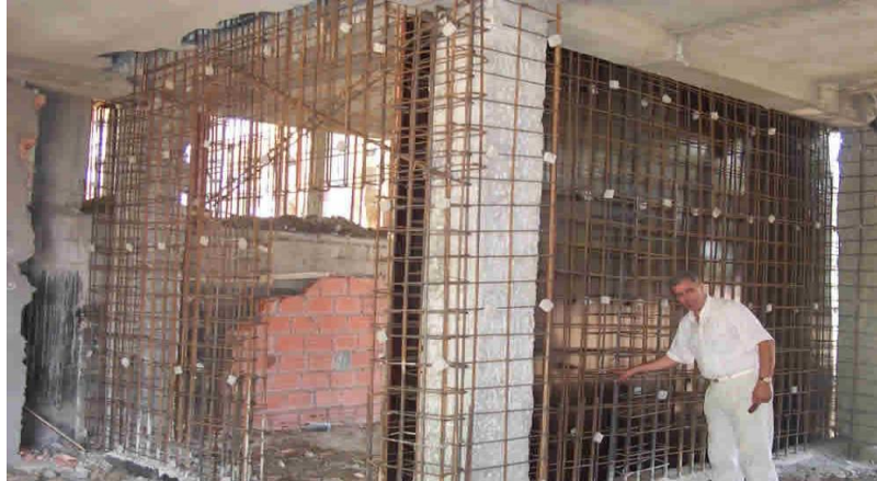
Fig 2.3 Retrofitting by adding shear wall.
