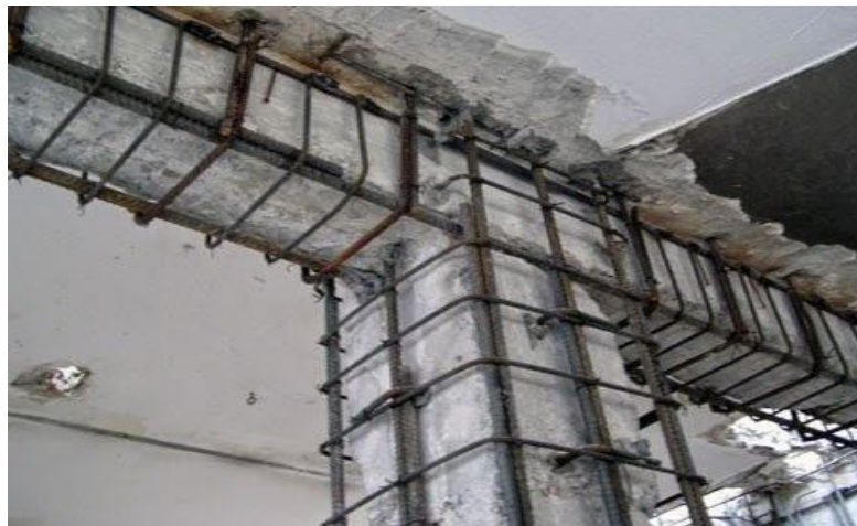
Fig 2.2 Concrete jacketing of beam and column joint.
