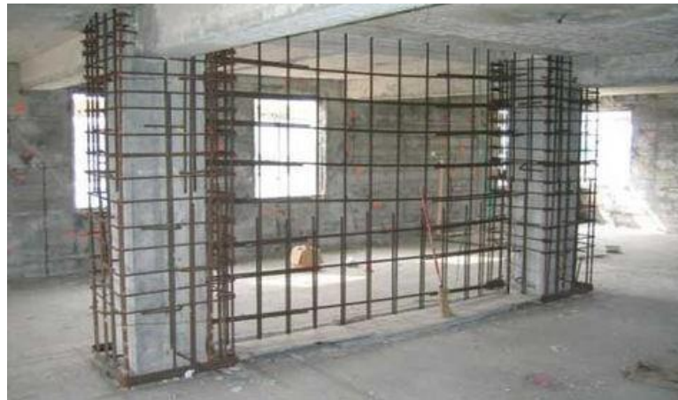
Fig 2.1 Process of concrete jacketing.
