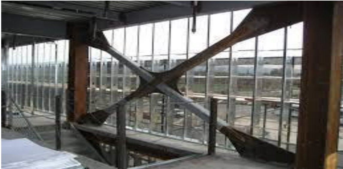
Fig. 1. 1 Inverted x Steel bracing
