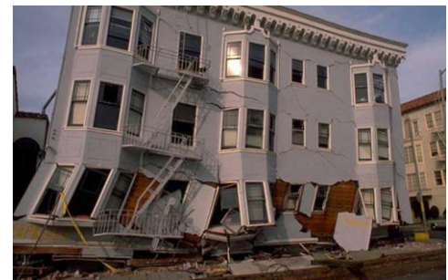
Fig1.2.2: Building collapse due to Earthquake
