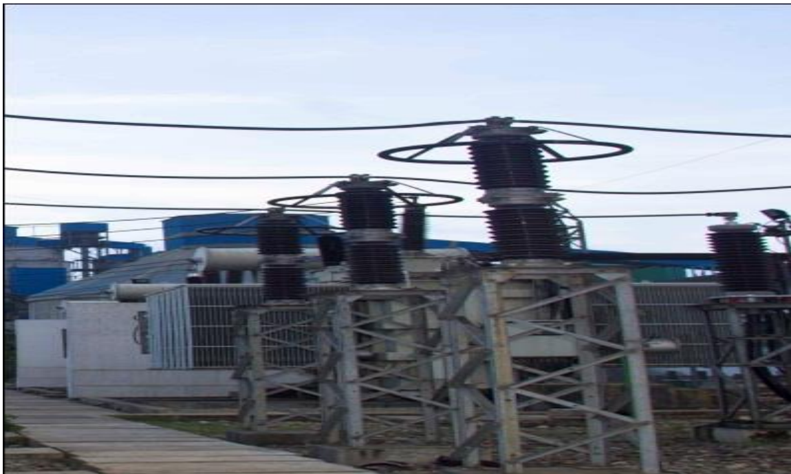
Figure 4.8: Lightning arrester
