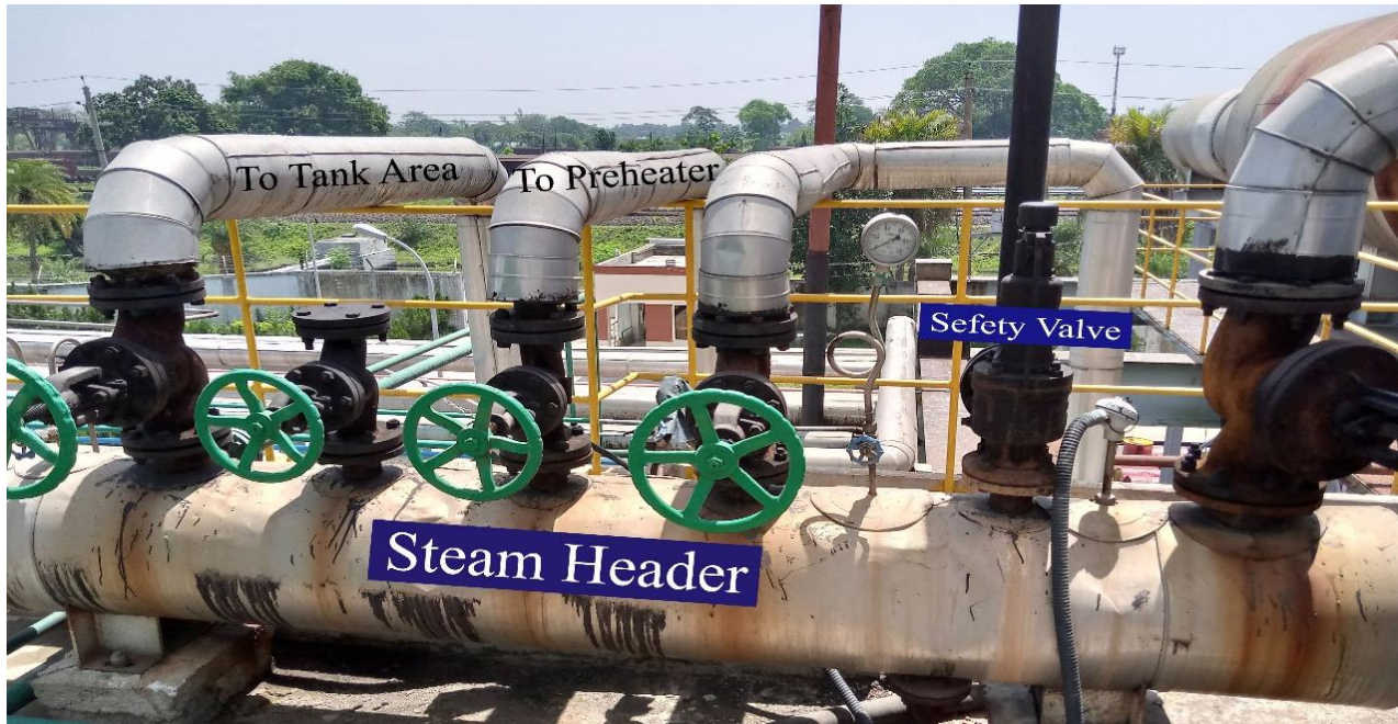
Figure 3.4 Steam Header
