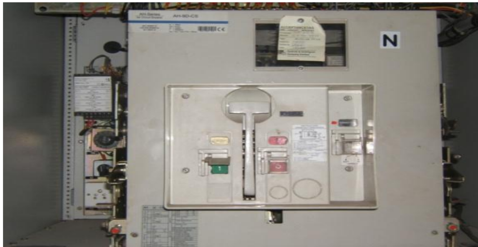
Figure 4.8: Air Circuit Breaker used in Santahar
