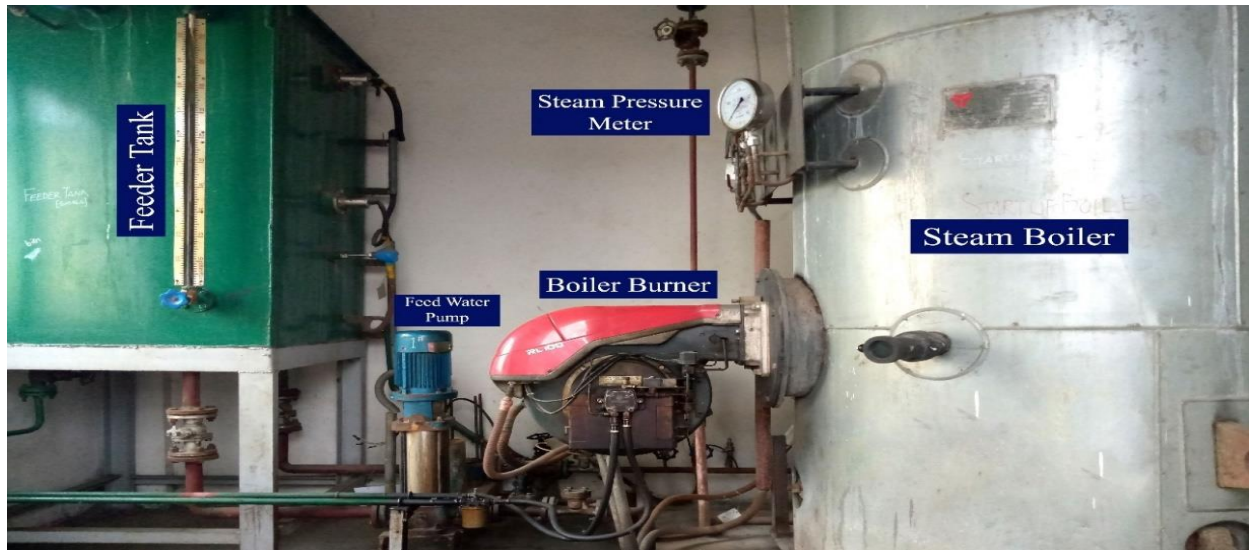
Figure 3.2 Startup Boiler
