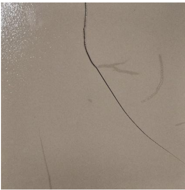
Figure 8 Crack tiles
