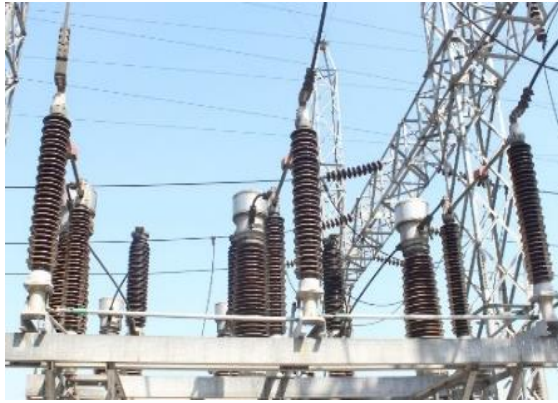
Figure 2.3: Lightning Arresters
