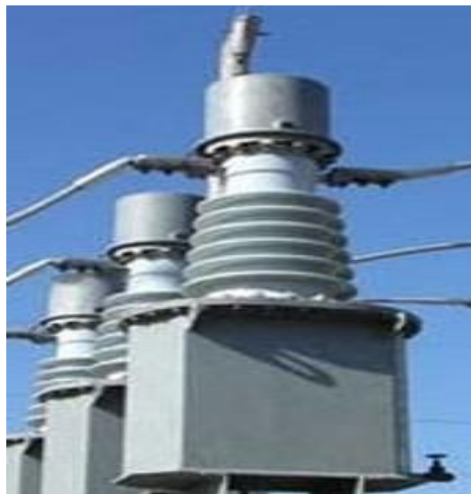
Figure 2.6: Current Transformer
