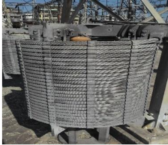
Figure 2.5: Wave Trap
