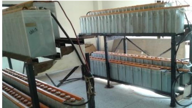
Figure 2.9: DC Power Supply
