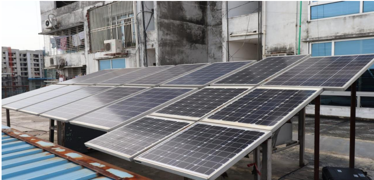
Figure 3.8: Working Place (To measure data)
