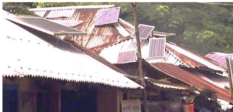
Figure 2.4: Solar home system in rural are
