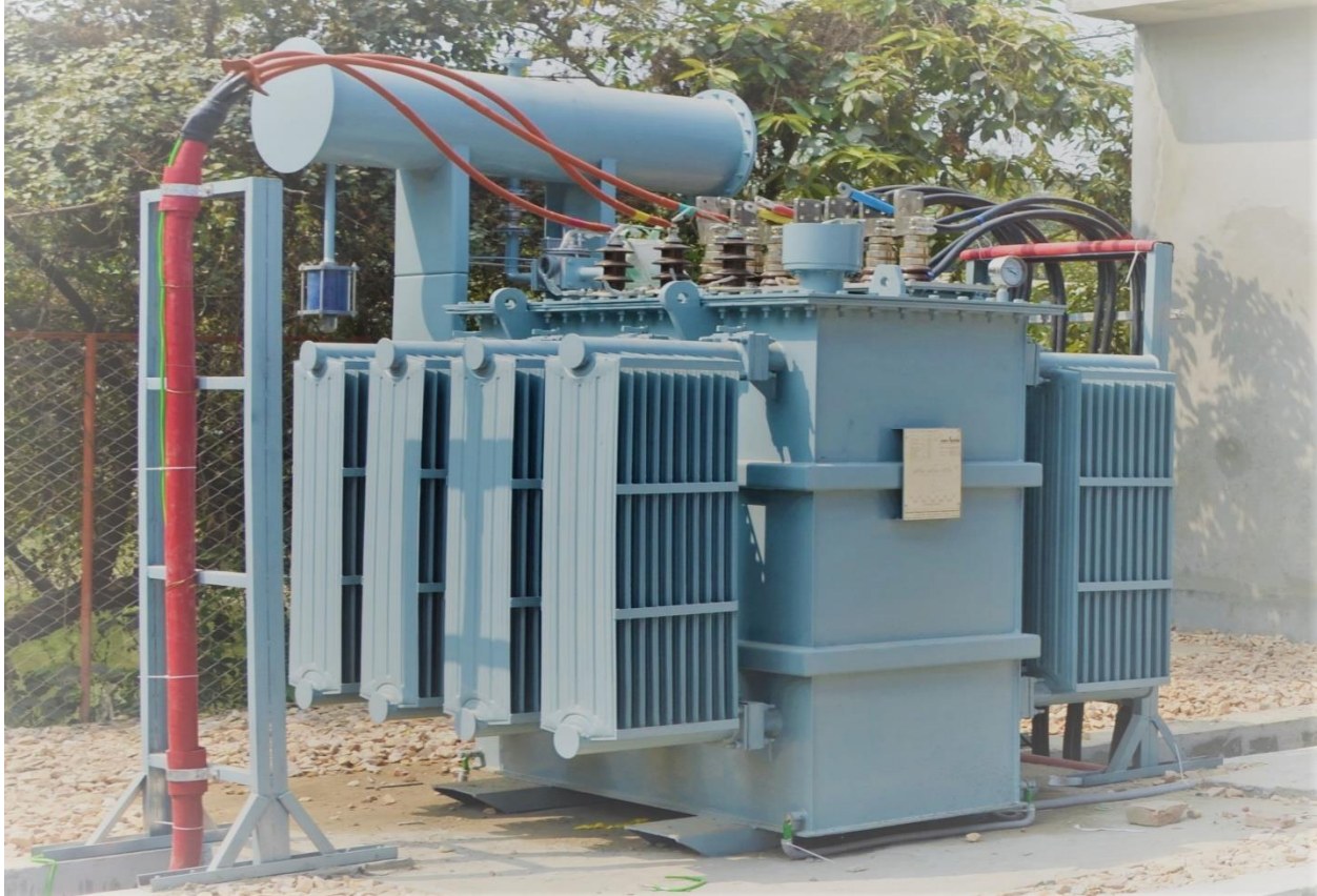
Fig 3.7 11/33 kv Transformer
