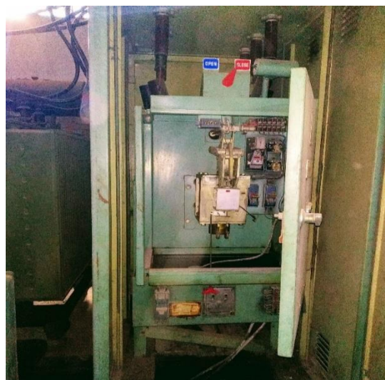
Fig 4.6 Vacuum circuit breaker
