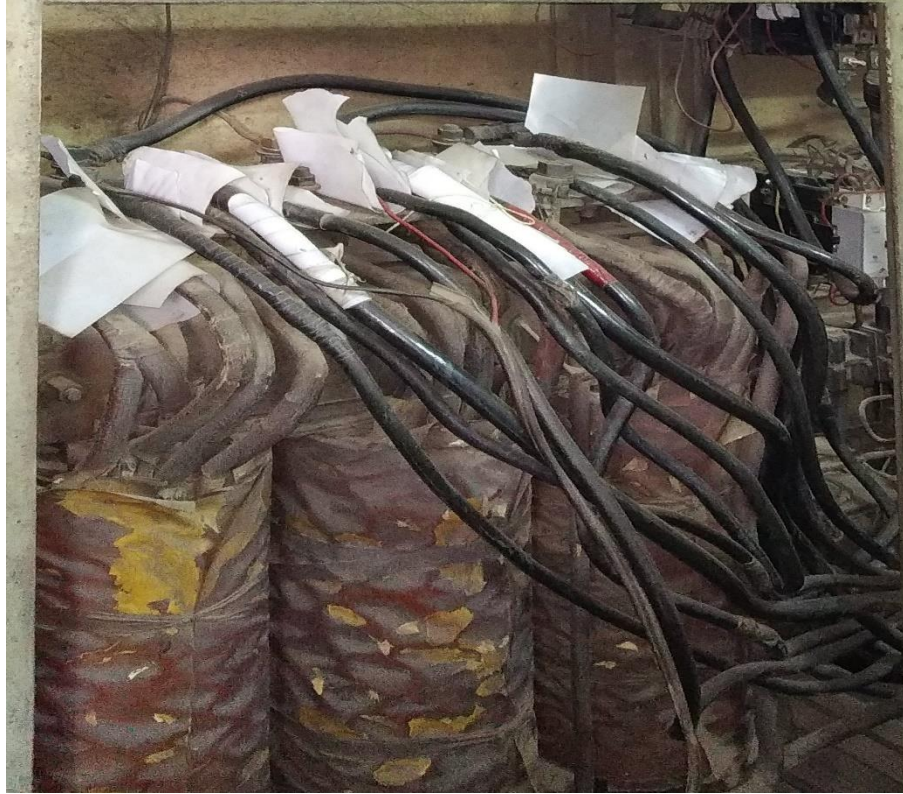
Fig 3.9 Transformer Winding
