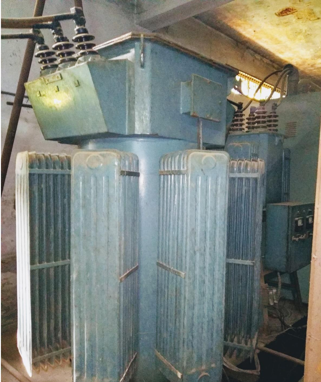
Fig 3.1 Distribution transformer
