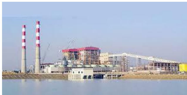
Figure 2.2: Steam Power Plant
