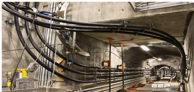
Figure 2.9: Underground Transmission Line
