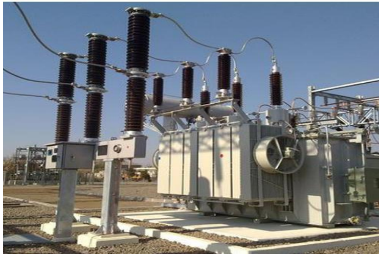
Figure 4.5: Power transformer
