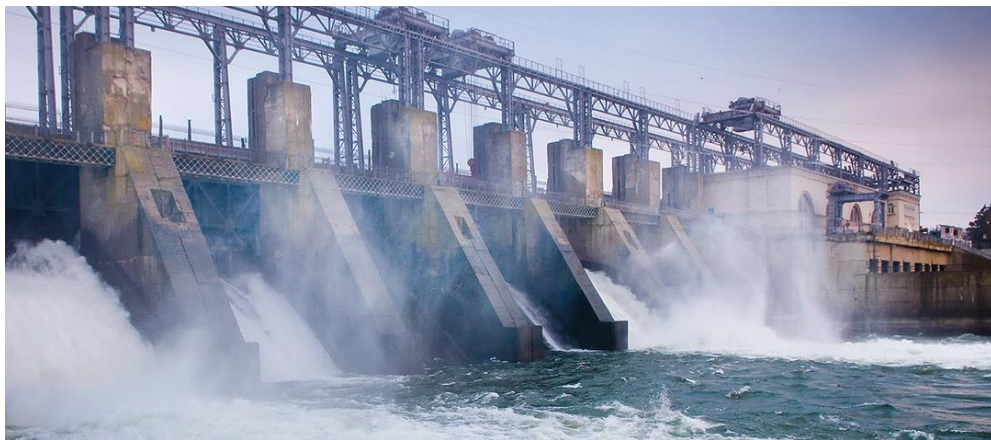
Figure 2.3: Hydro Electric Power Plant
