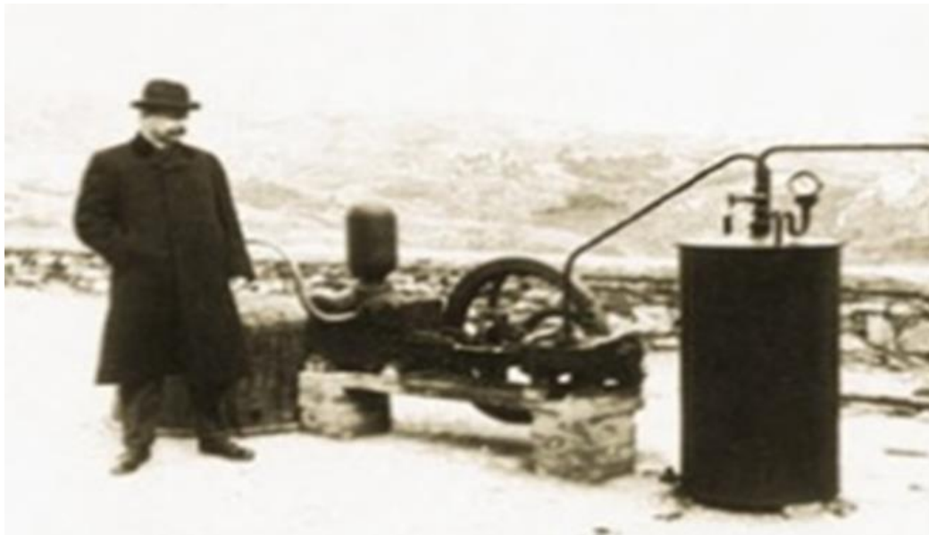
Figure 1.2: First Geothermal Power Plant in Larderello. Italy
