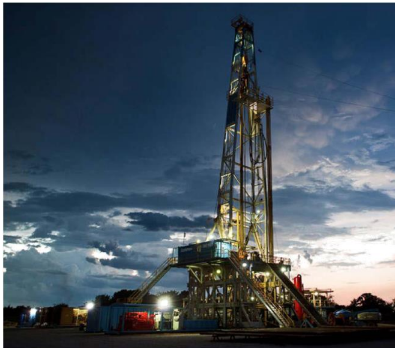
Figure 4.13: Typical Land Conventional Rig [10]
