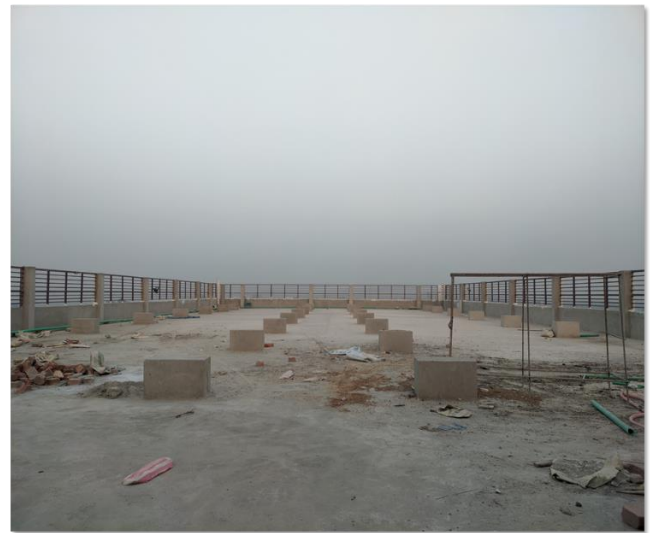
Fig.3.5: East side rooftop view
