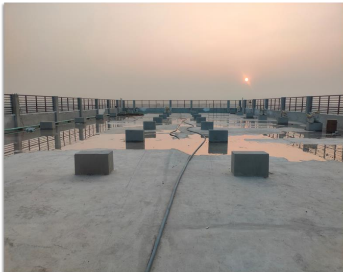
Fig.3.4: West side Rooftop view
