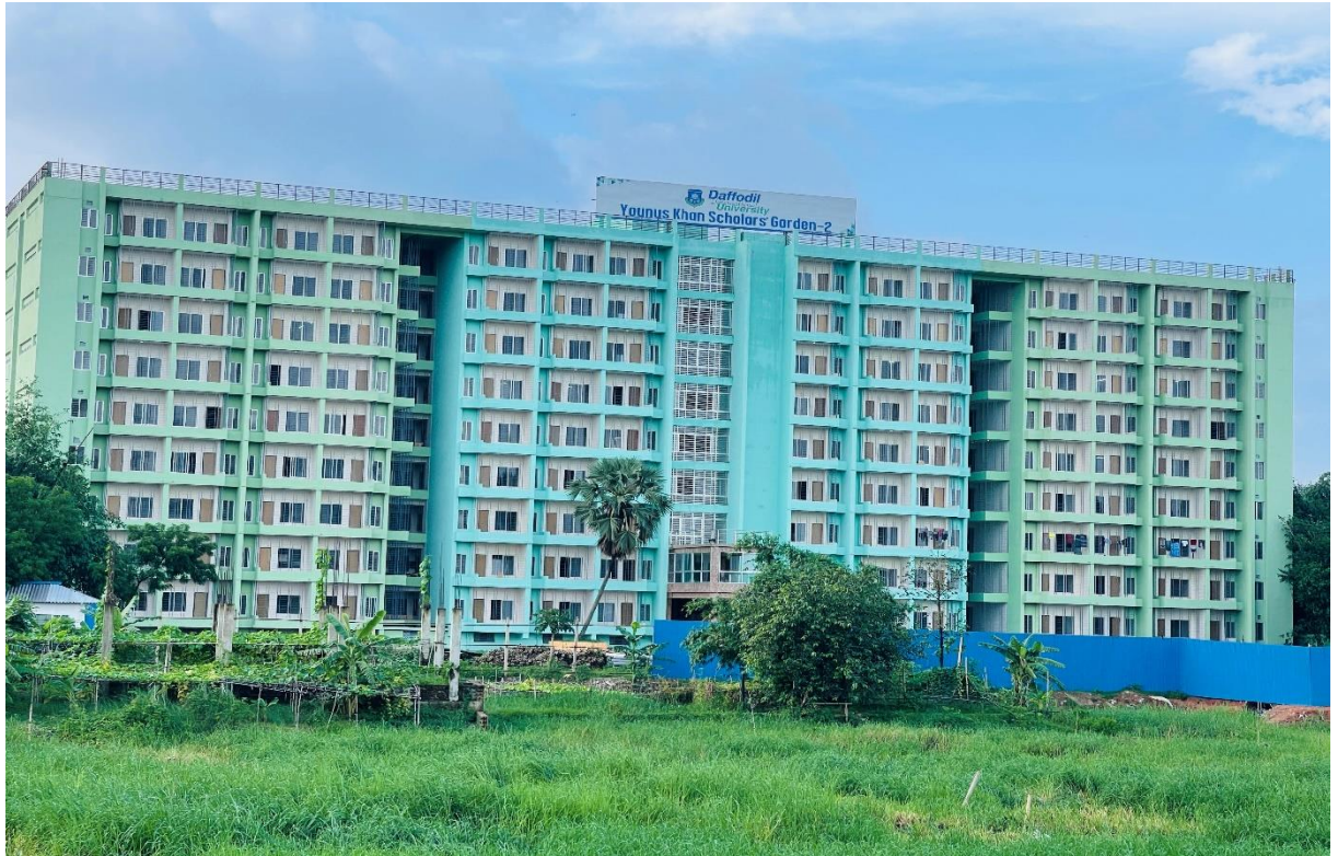
Fig.3.3: Building Site Front View
