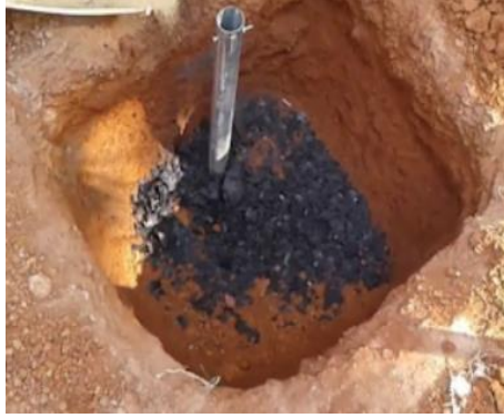
Figure: 2.16: pipe earthing
