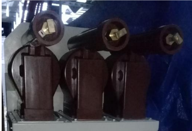
Figure: 2.8: Potential transformer (PT)
