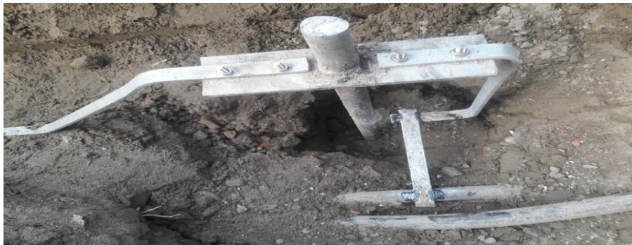
Figure: 2.17: Rod earthing
