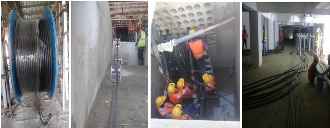
Figure: 3.1: underground cable laying
