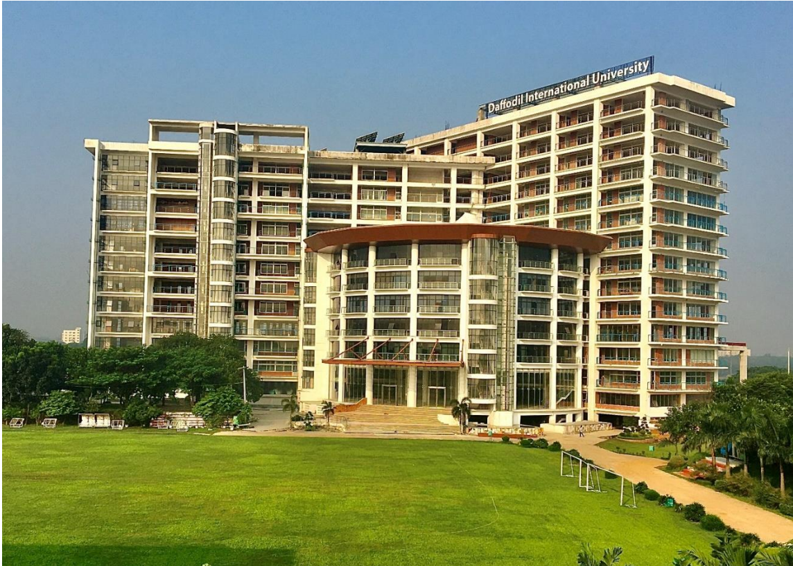
Figure 6.1: Front view of Academic Building 4
