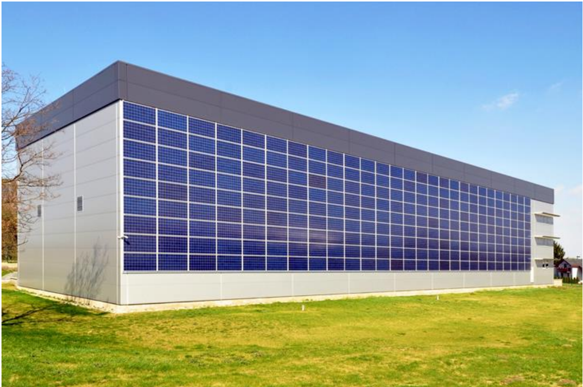
Figure 5.5: Building Integrated Photovoltaic [35].
