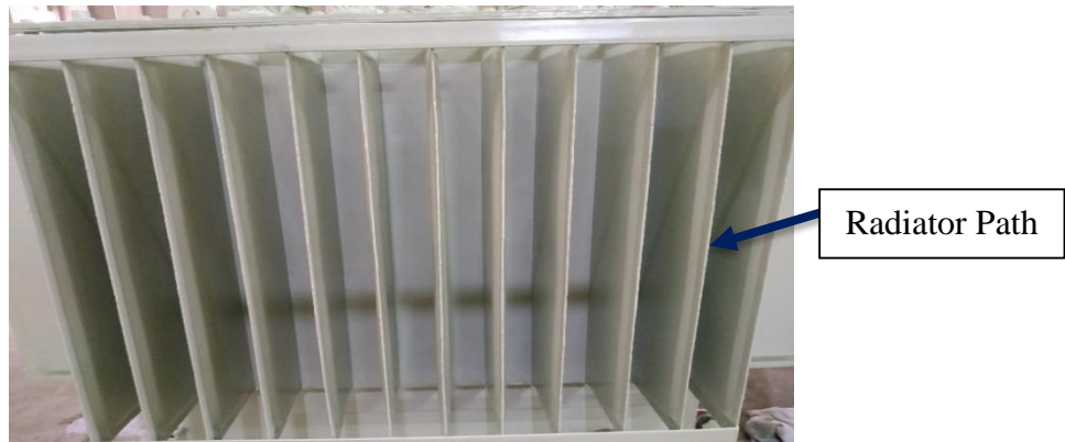
Figure 3.12: Transformer Radiator
