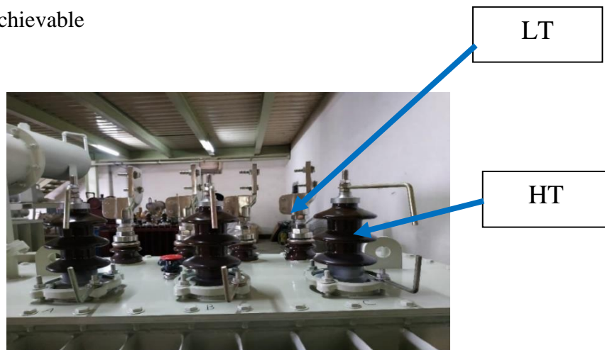
Figure 3.7: HT and LT Bushing
