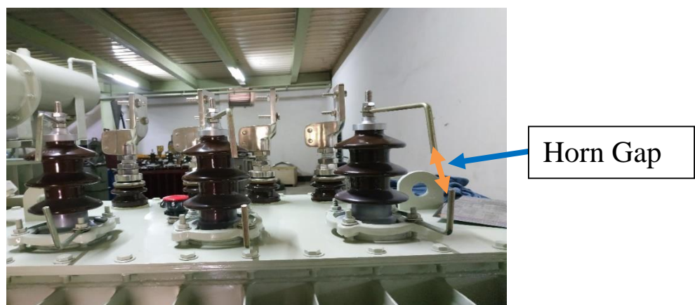
Figure 3.17: Horn Gap
