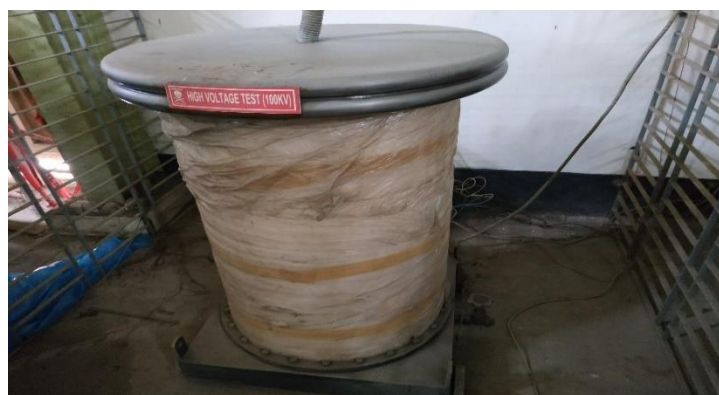
Figure 5.7: High Voltage Test
