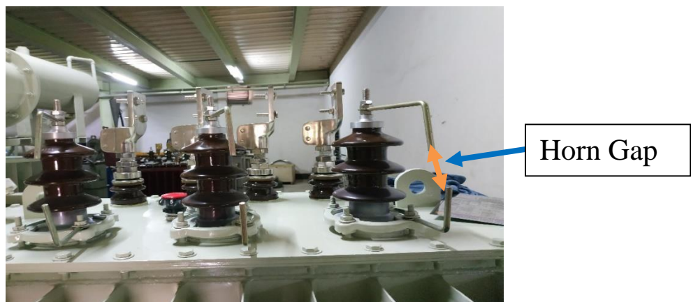
Figure 3.17: Horn Gap
