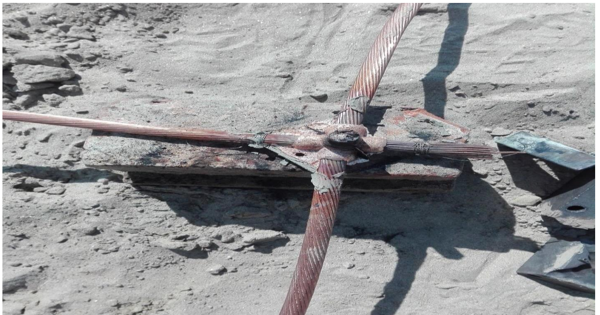
Fig. 4.3 Joint of sub mass with main mass in Rajendrapur 132/33 KV grid substation
