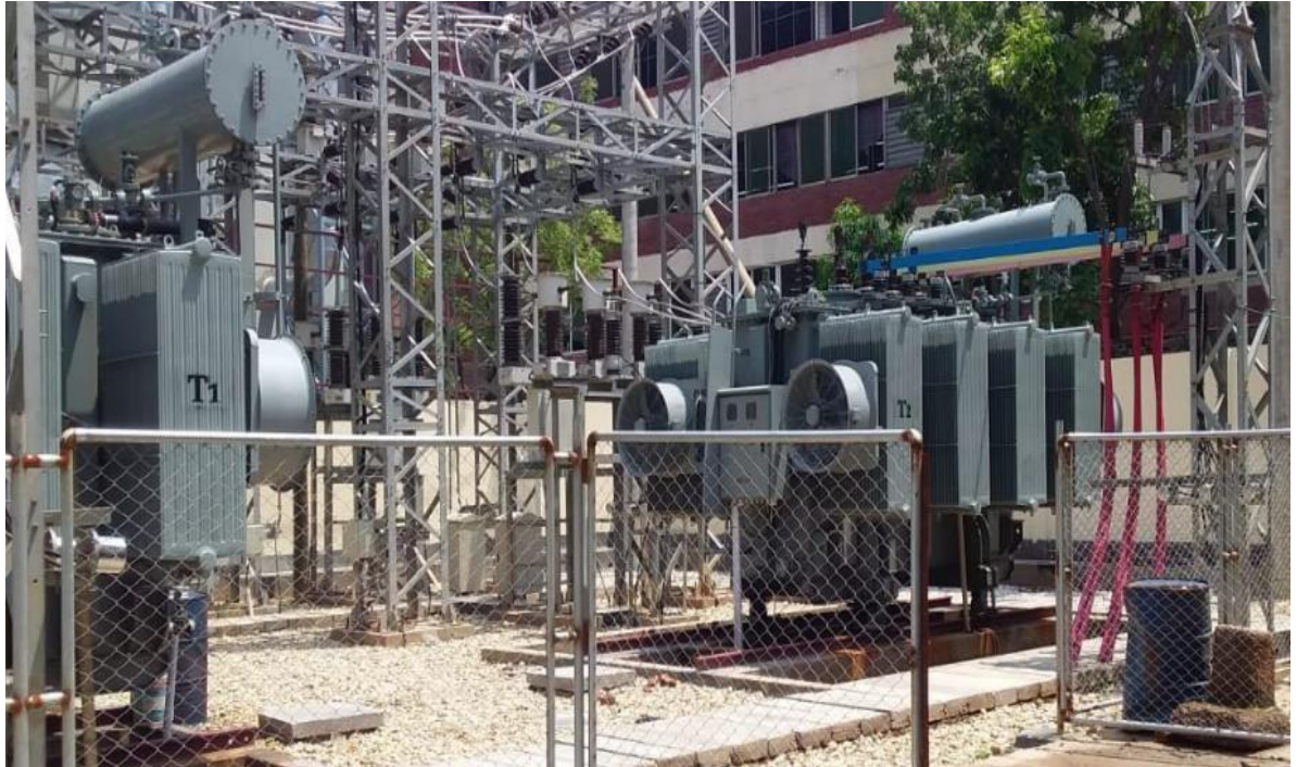
Fig. 2.5 Distribution Substation
