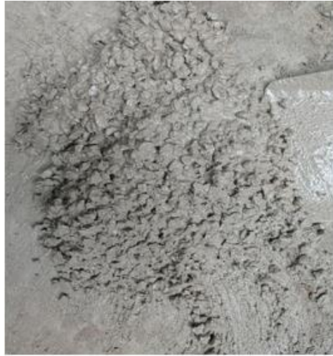
Figure 3.7: Mixing concrete (Mixing by hand)
