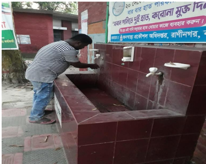
Figure-2.1: Pictures of Sanitization Process in Naogaon Raninagar upazila office.
