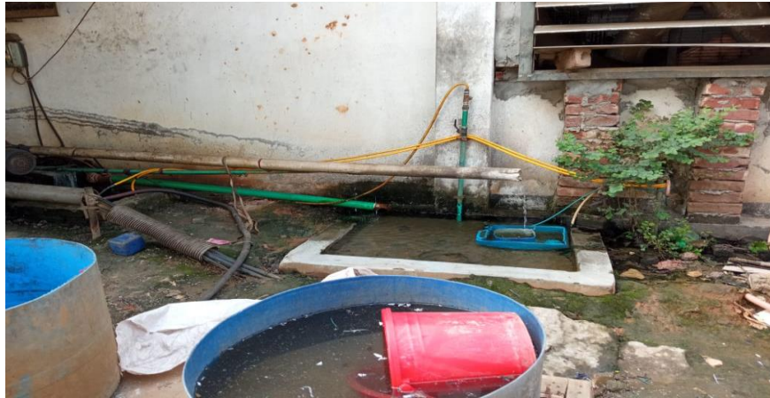
Garments are leaking dirty water.
