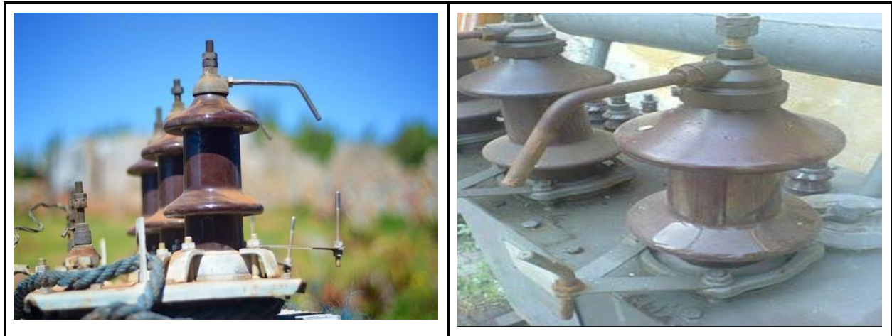
Figure 4.4.8 Horn Gap
