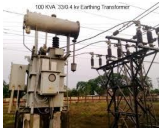
Figure 4.6.1 Transformer Earthing
