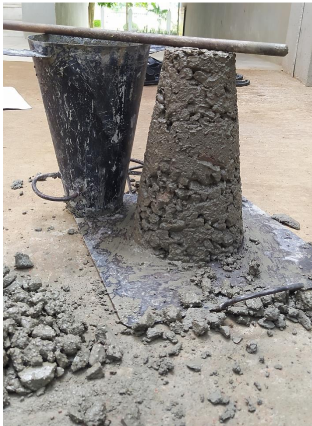
Figure 3.3: Concrete Slump Test and Observed
