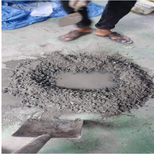
Figure 18: Mixing Stone sand cement and water in concrete
