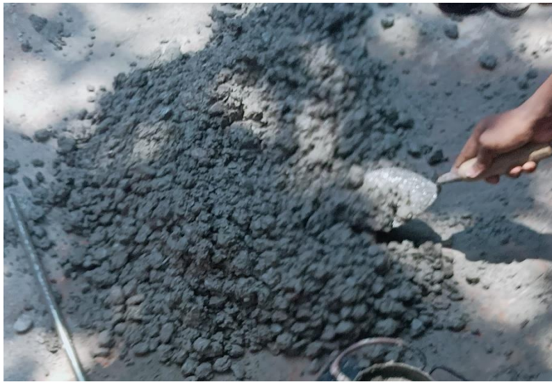
Figure 3.6: Concrete mixing
