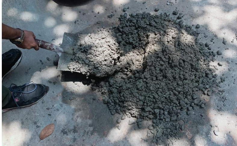
Figure 2.2: Hand mixing of concrete
