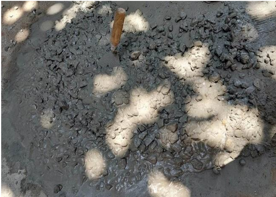
Figure 3.6: Mixing Concrete (Hand Made)
