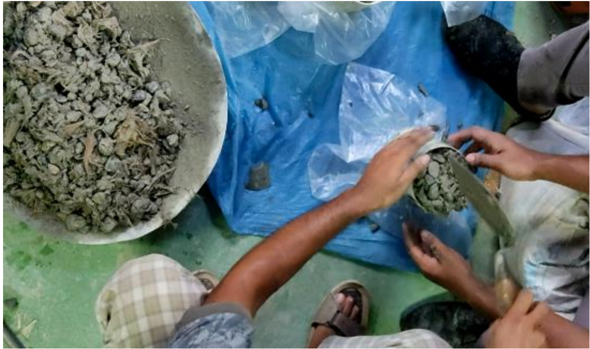
Figure 0-11: Casting the mould with concrete
