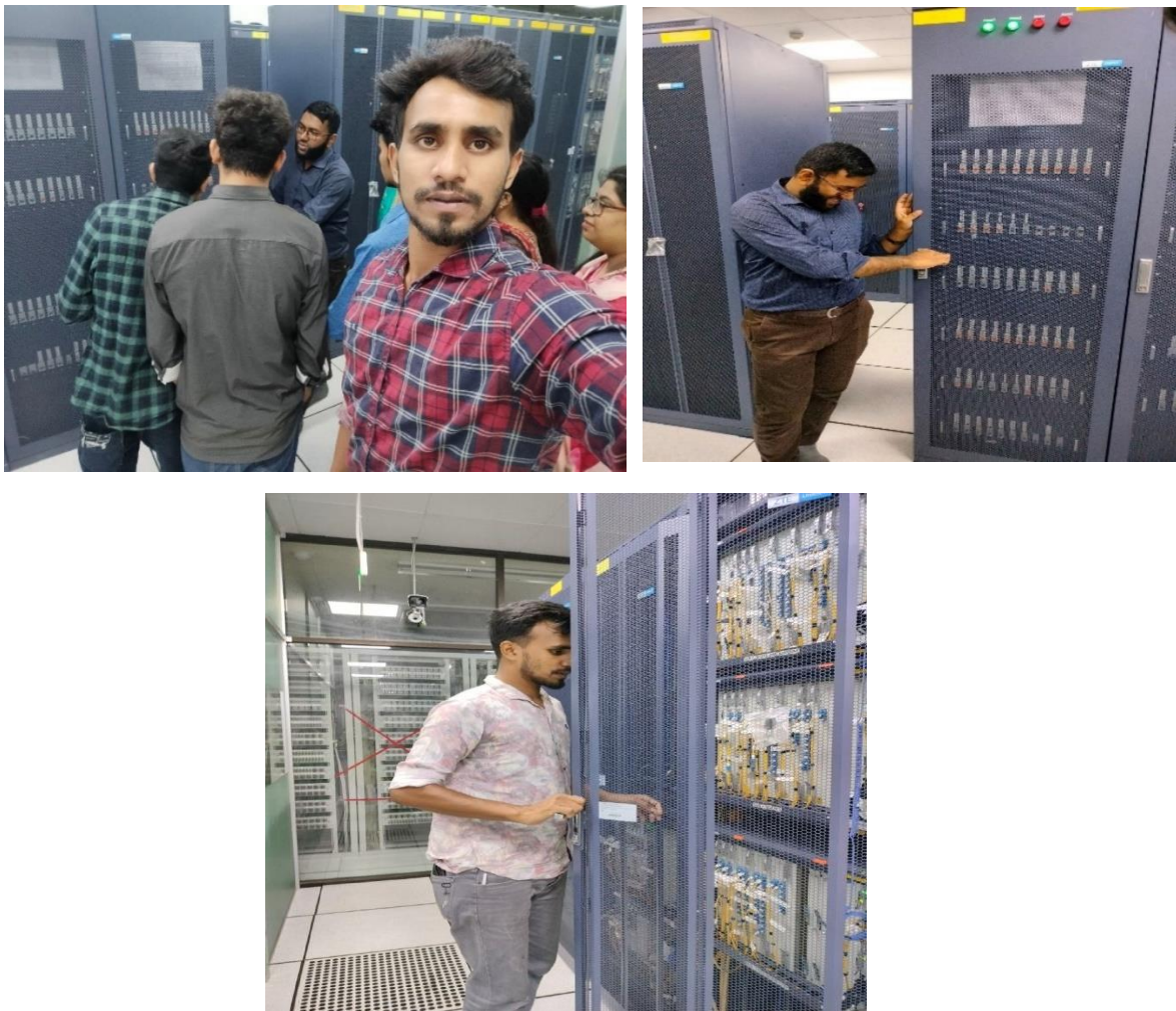
Fig 5.5: Working time in the switch room
