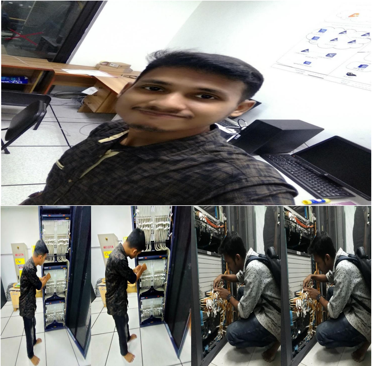
Figure 4.1.1: working in switch room
