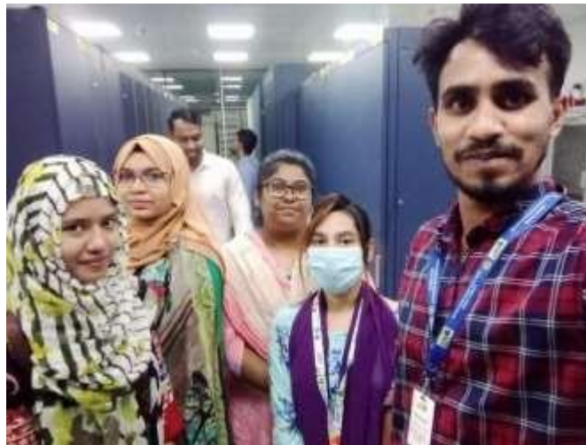
Figure 3.1 Working at Switch Room with my Group Member
