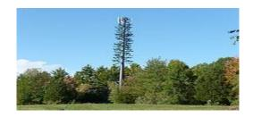
Fig 6.4 Cellular antenna disguised to look like a tree
