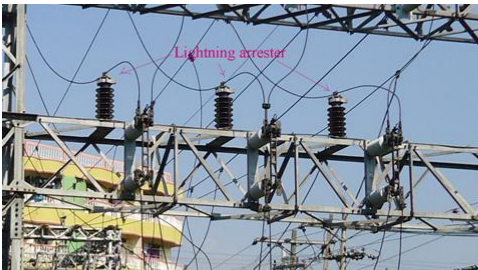
Fig 6.11: Lightning arrester
