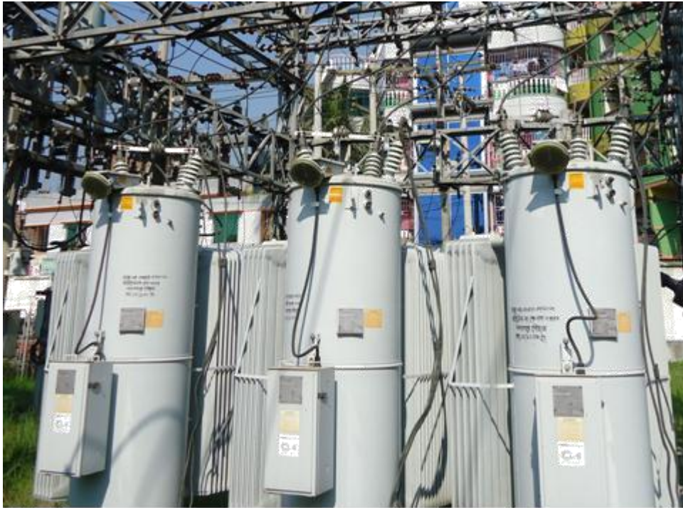
Fig 6.13: Voltage regulator
