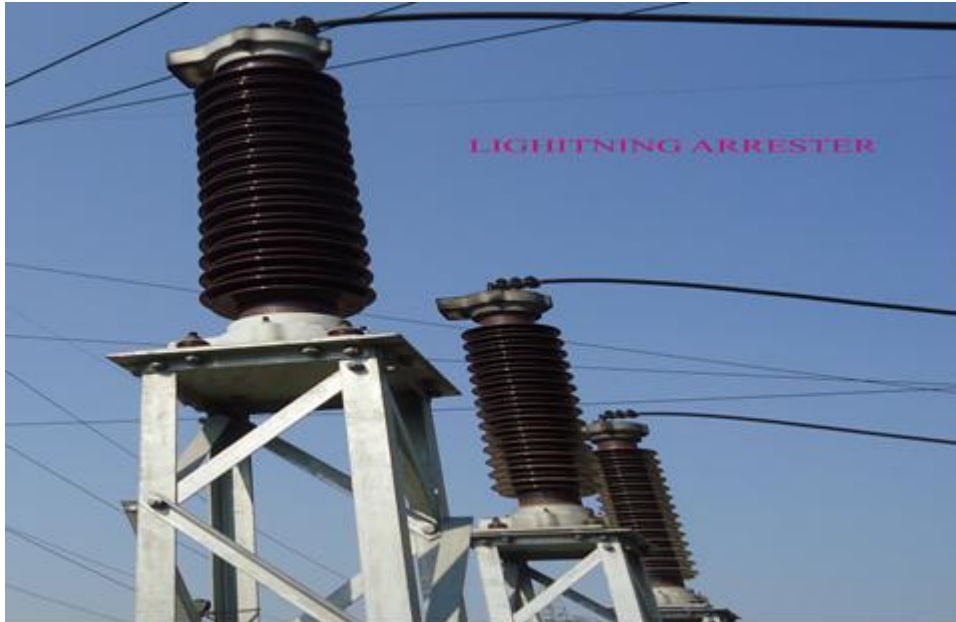
Fig 8.7: Lightning Arresters
