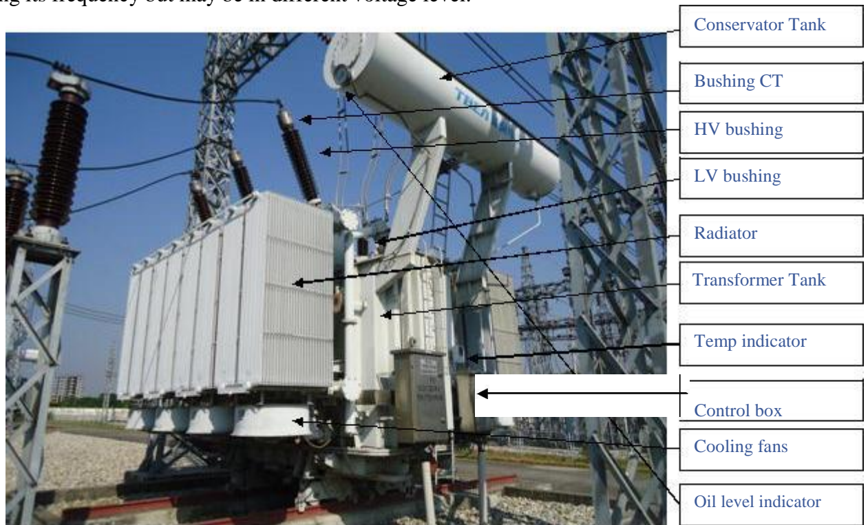
Fig 8.10 : Power transformer
