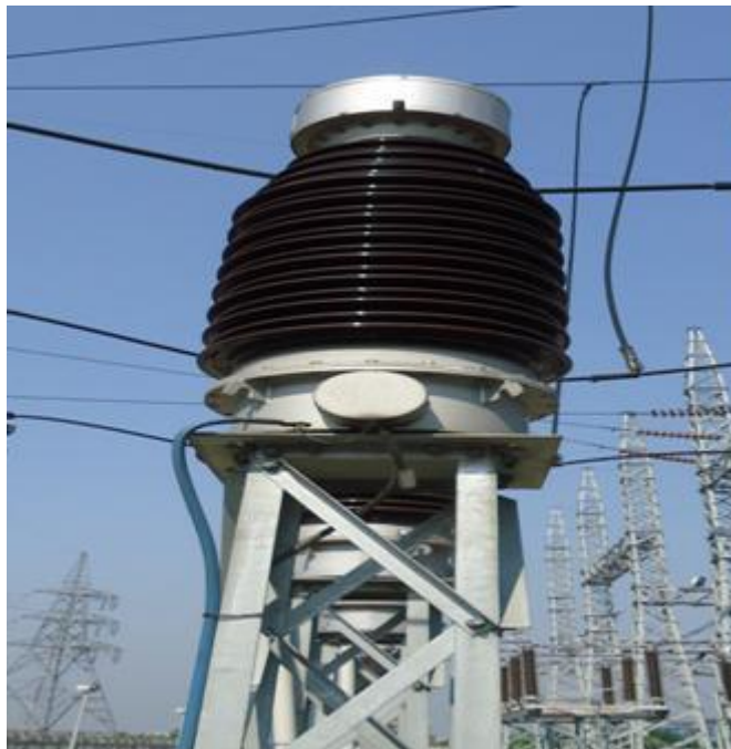
Fig 8.3: Potential Transformer
