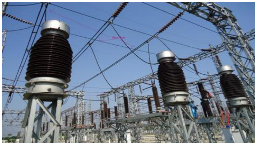
Fig 8.9: Bus-bar arrangement
