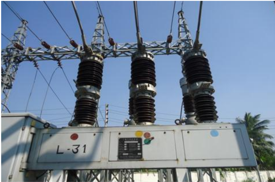
Fig 7.3: Automatic Circuit Recloser (ACR)
