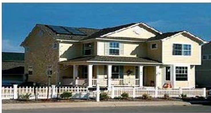
Figure : The family living in this house enjoys hot water heated by the sun with a solar thermal system
