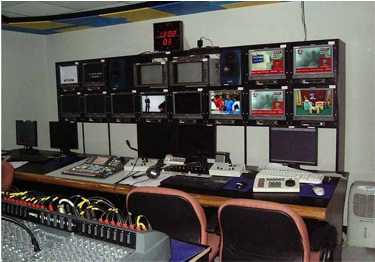
Figure 3.2 inside the Production Control Room (PCR)[1]
