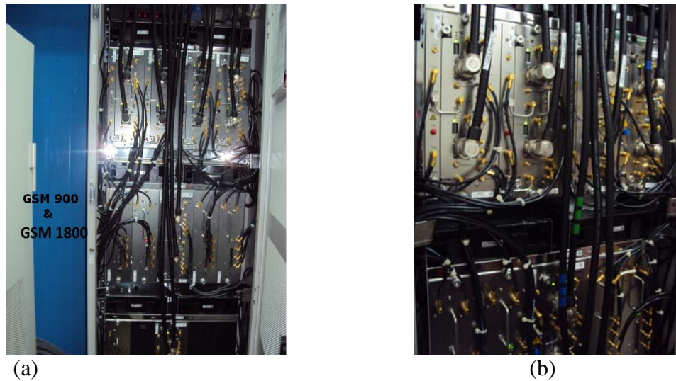
Figure 6.3: (a) Duel Band BTS cabinet (b)TX & RX connection and Antenna cables
