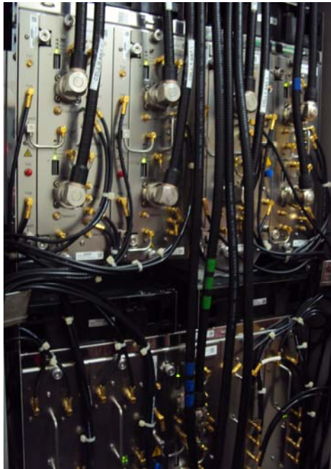
Figure 3.5: Flexi CU EDGE- a doubled capacity transceiver that supports EDGE by Teletalk
