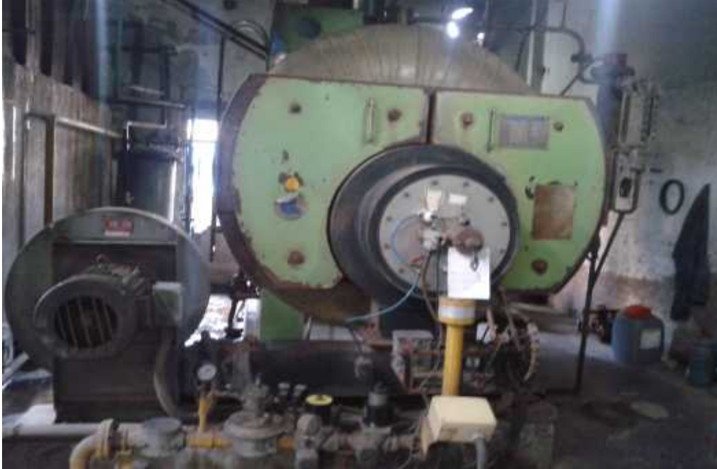
Fig: Cochran Boiler, Fire Tube
