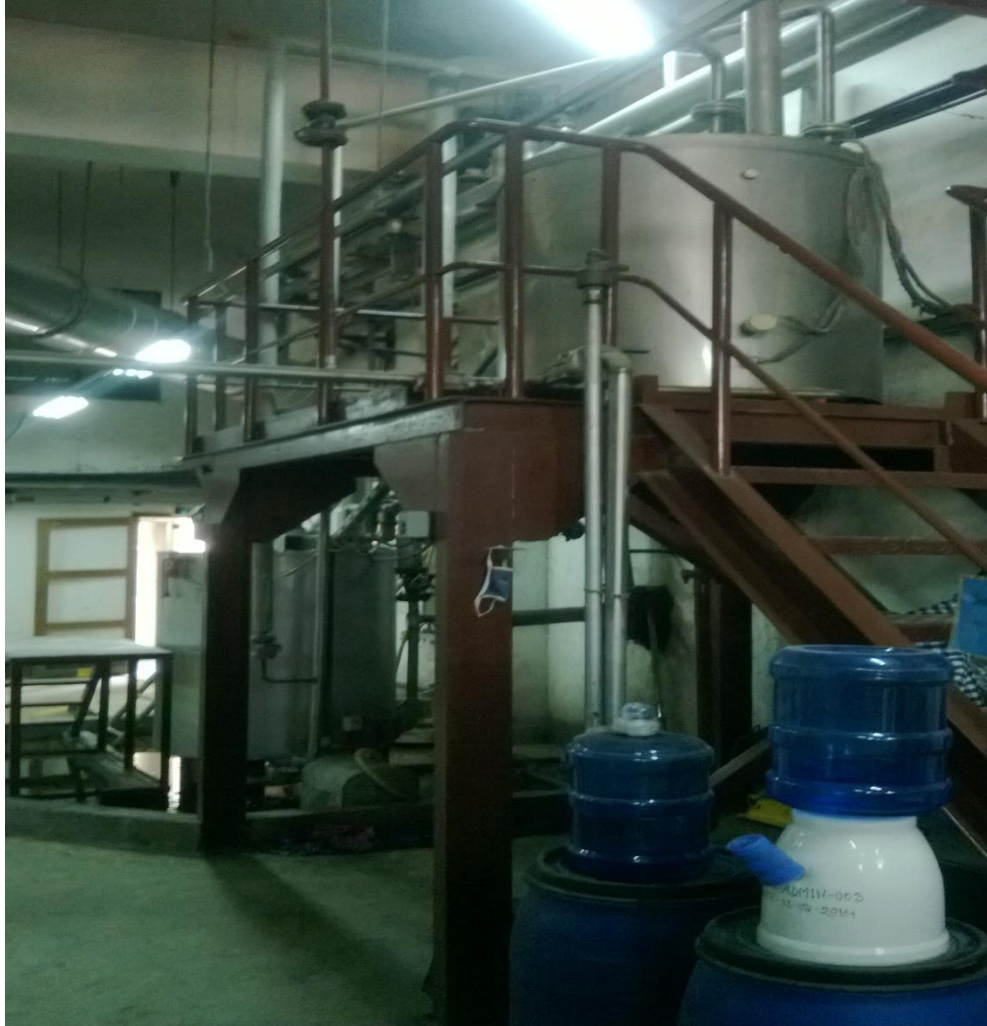
Fig: Sizing Tank
