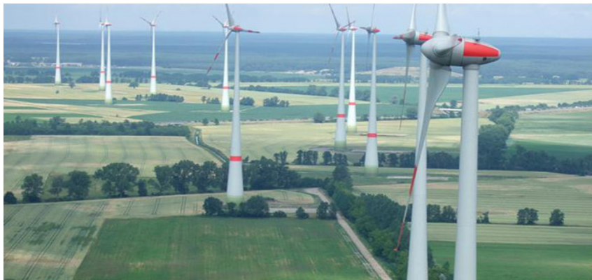
Fig: 6.1 Wind turbine connections in wind farm
