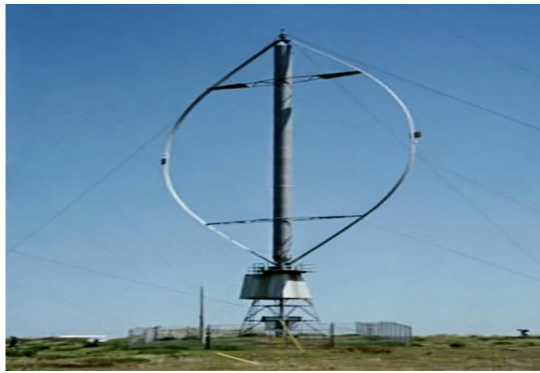
Fig:1.8 Vertical axis wind turbines – Darrieus type
