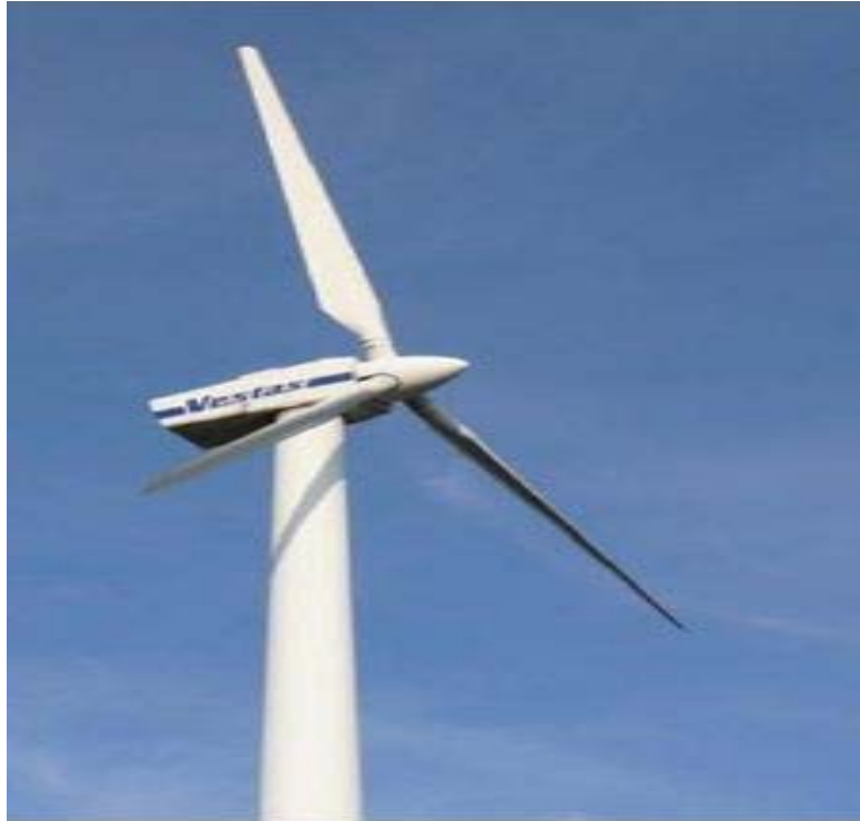
Fig:1.3 Horizontal axis wind turbines (3 bladed wind turbine by vestas, a Danish company that make large wind turbine, from 0.85MW to 3MW.)
