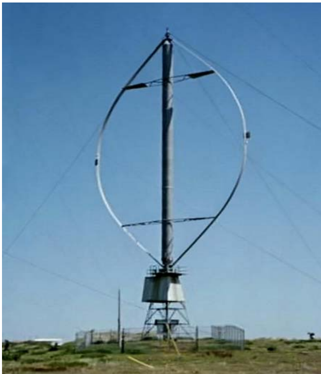
Darrieus Wind turbine with classic tropsokein or egg-beater shaped rotor. This one features a 30 meter high rotor.
