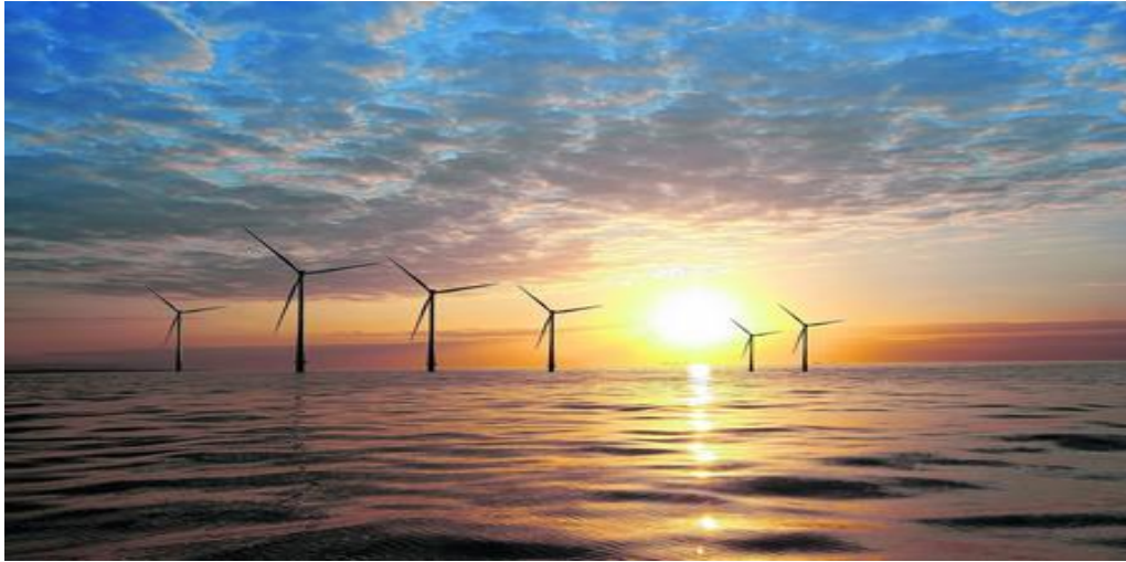
Fig: 5.3 Offshore Wind Farm
