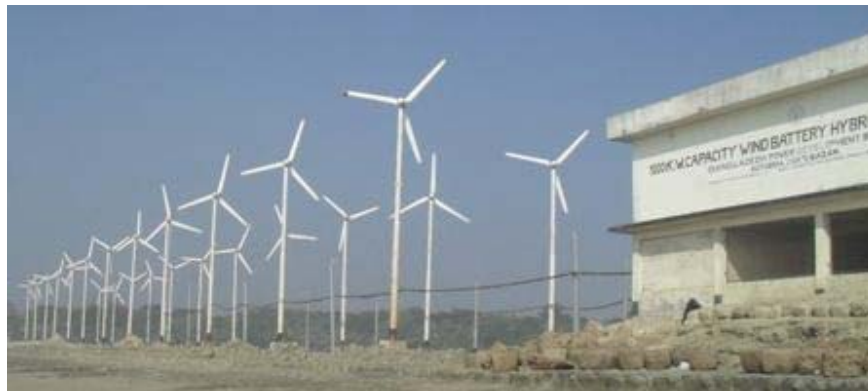
Fig:8.2 1000KW Wind Battery Hybrid Power Plant (so called Light House)
