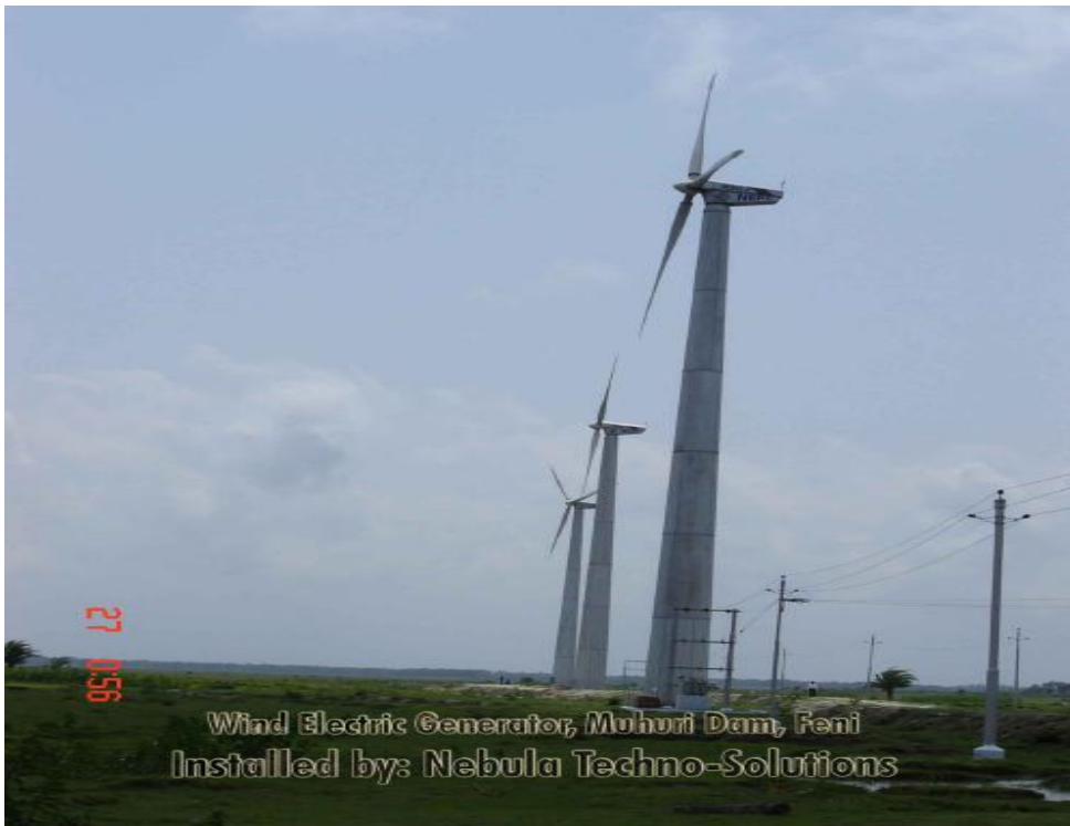
Fig:8.5 900kw grid connected of Muhuri dam
