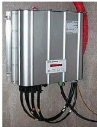
Fig21: Inverter for grid connected PV
