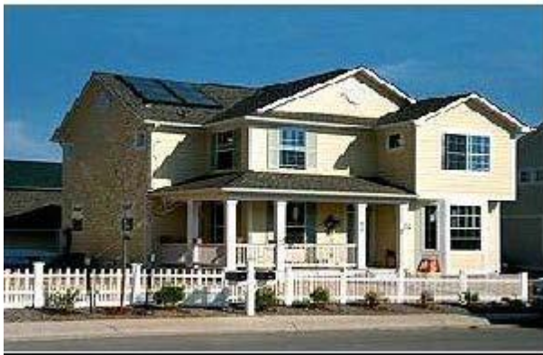
Fig2: The family living in this house enjoys hot water heated by the sun with a solar thermal system
