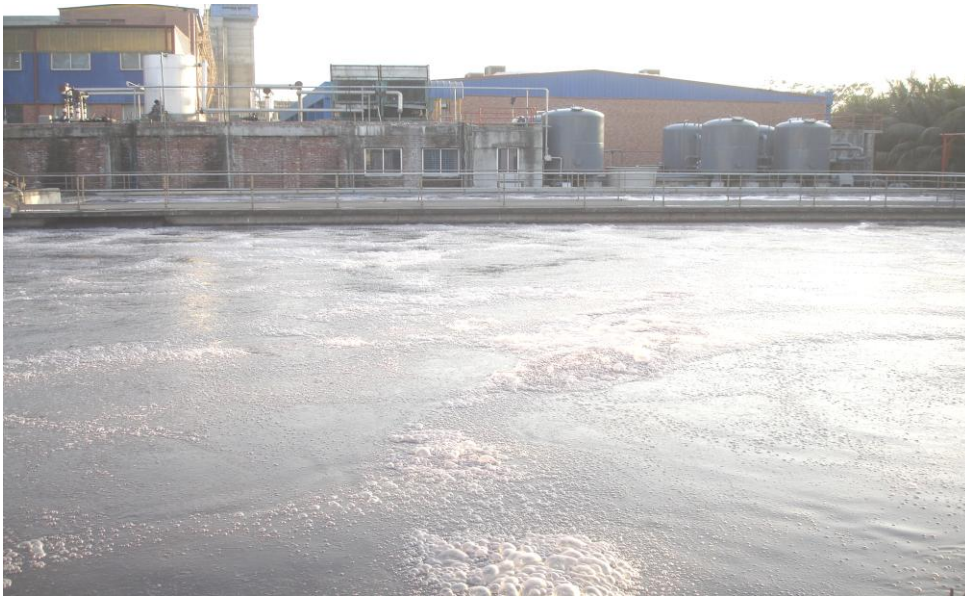
Effluent Treatment Plant
