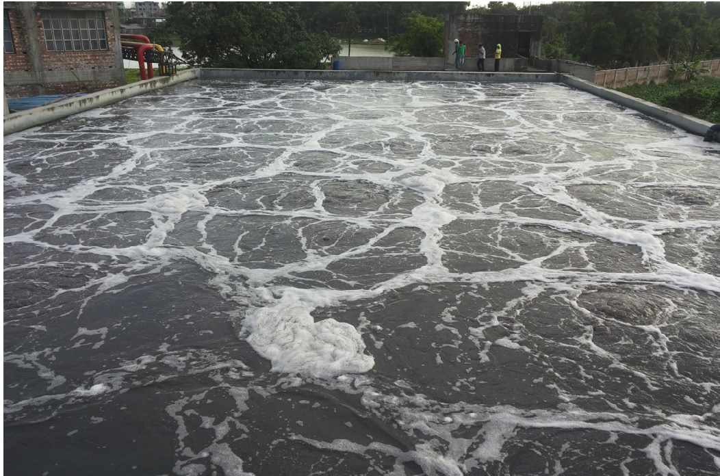
Figure 4.8: Ecolization tank at DFL
