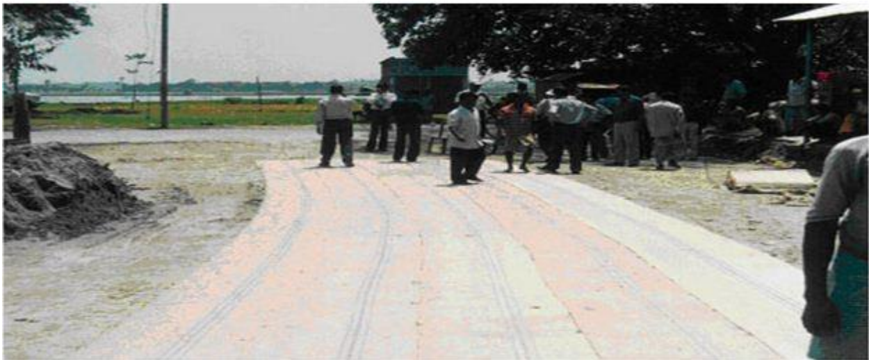
Figure: use of jute geo-textile in road
