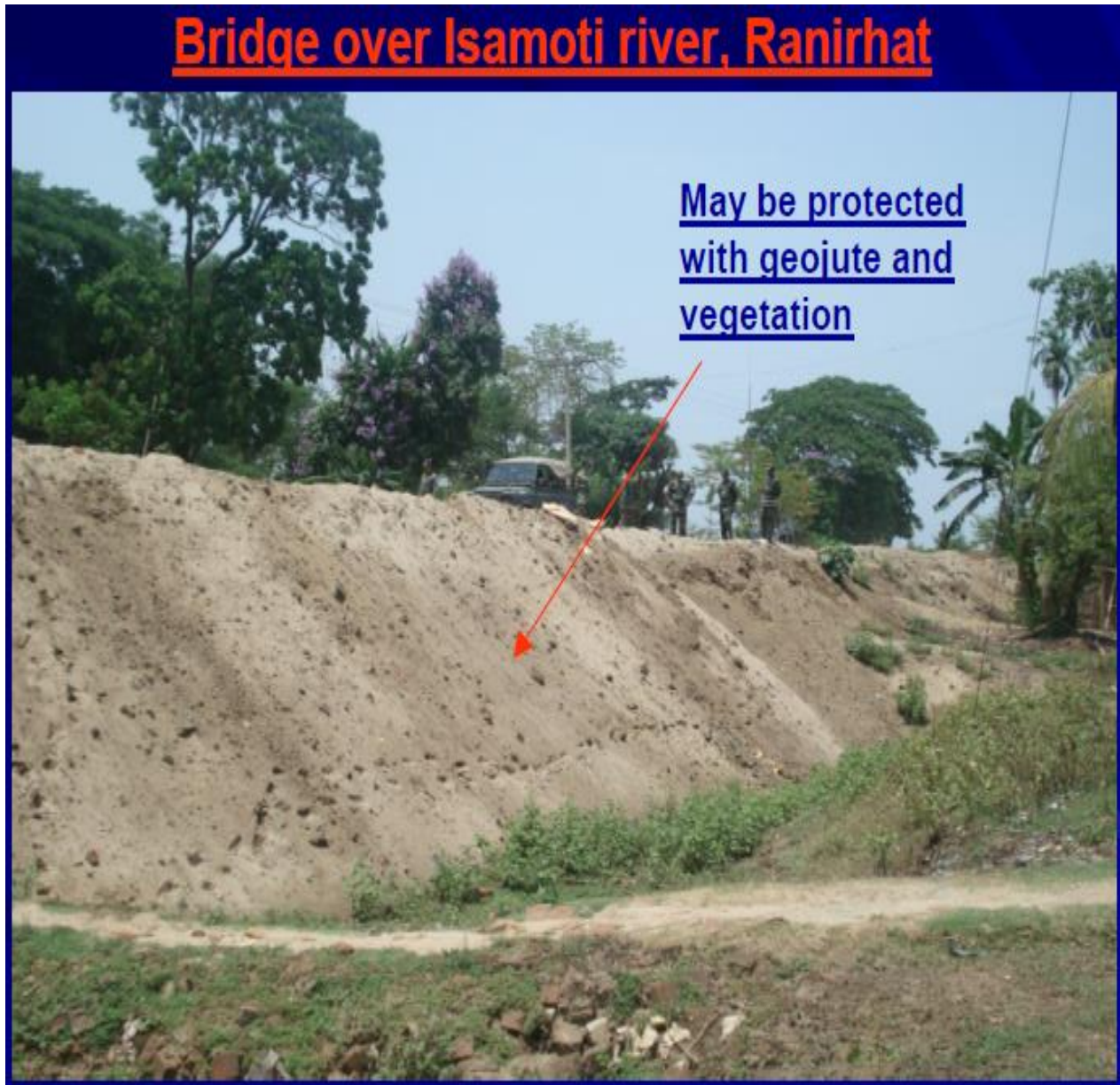
Fig: Slope and Wall Reinforcement
