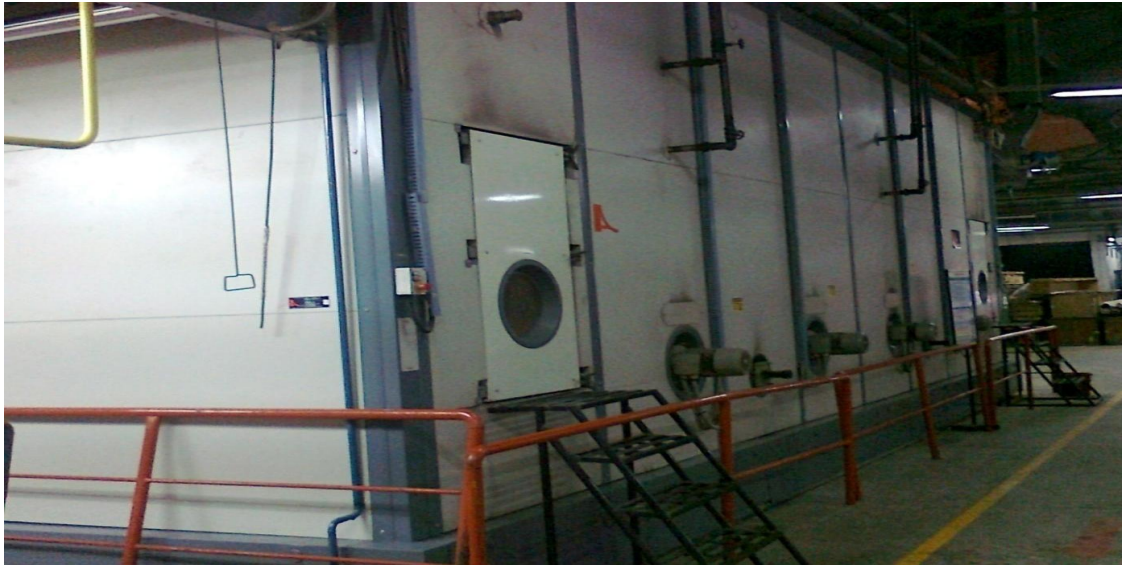
Fig: Curing Machine
