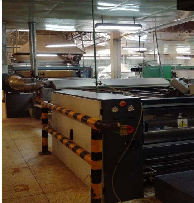
Fig: 3.16 Compactor machine
