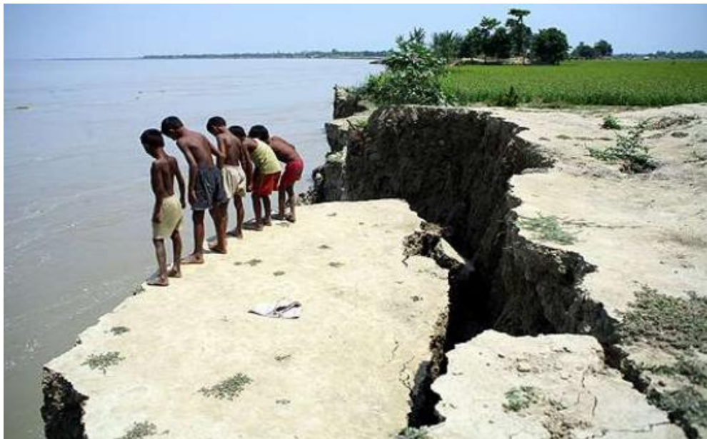
Figure 11: Photograph of River Bank Erosion
