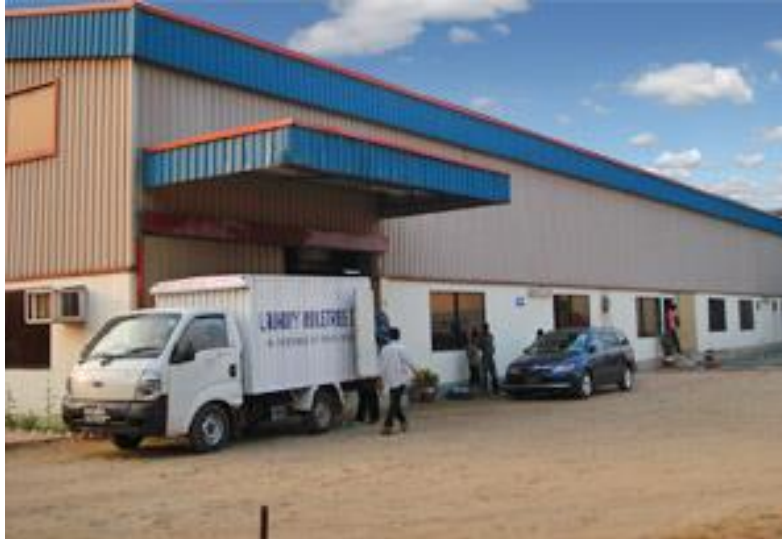
Fig 3.8.1: Front view of Laundry
